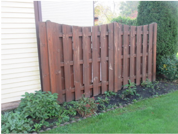
Typical wood privacy fence perpendicular to unit rear elevation
