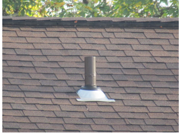
Example of rubber seal with metal base boot flashing at waste pipe penetration of asphalt shingle roof
