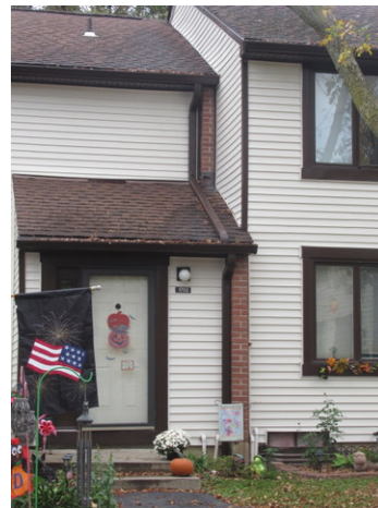
Aluminum gutter and downspout overview
