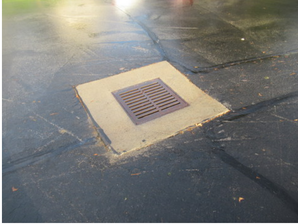
Typical catch basin
