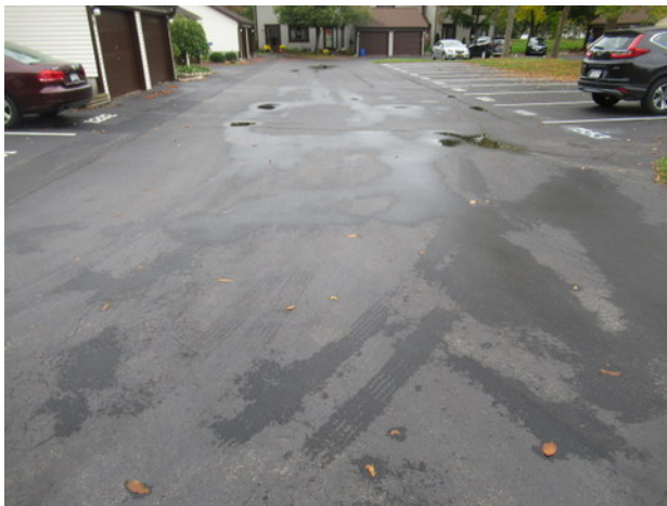
Asphalt pavement overview (typical street and parking area)
