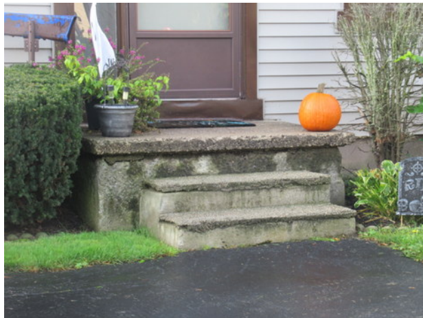
Typical front entrance stoop
