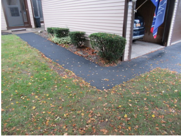
Asphalt pavement overview (typical walkway between front entrance and driveway)
