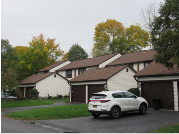
Asphalt shingle roof overview
