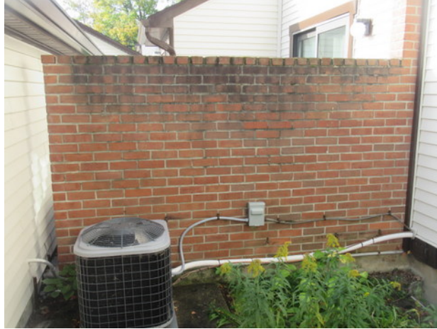
Typical masonry privacy wall
