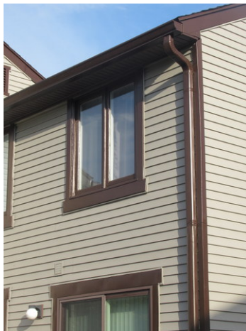
Aluminum gutter and downspout overview
