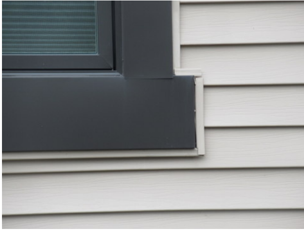
Example of J-channel at interface of vinyl siding/window
