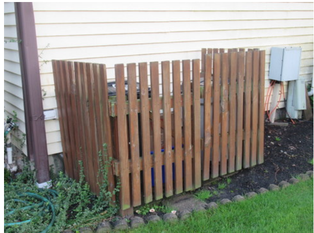
Typical wood refuse area fences located at the side elevation of building
