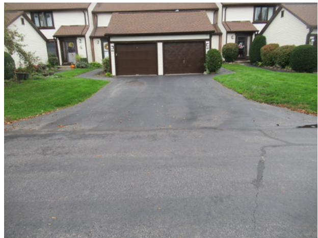
Asphalt pavement overview (typical driveway)
