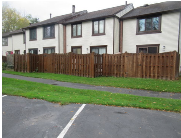
Example of wood privacy fences parallel to unit rear elevations
